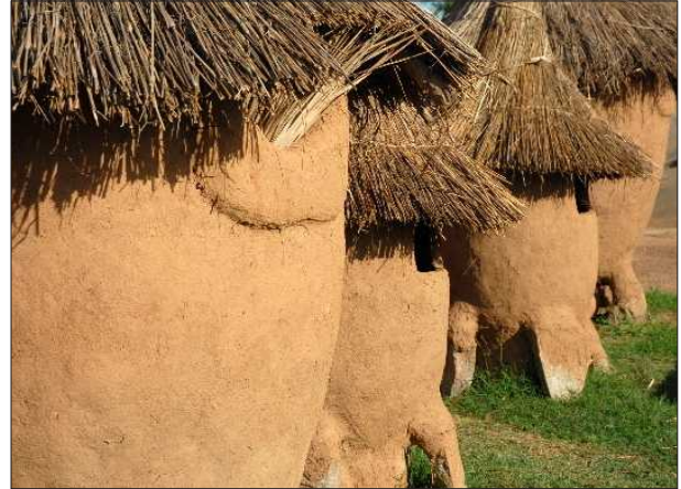
Mud cow dung coated bamboo based food grain storage
